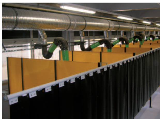
General views of welding booths built with partition steel panels in training welding center
